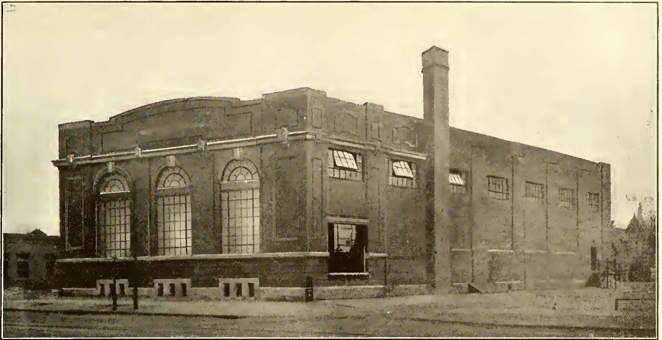
A TYPICAL HIGH-GRADE SUBSTATION BUILDING—CEDAR AVENUE SUBSTATION, CLEVELAND (OHIO) RAILWAY
