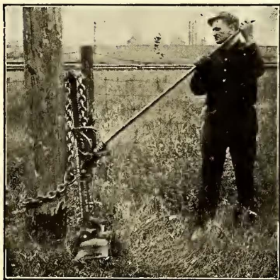
USING A JACK TO RAISE A POLE
