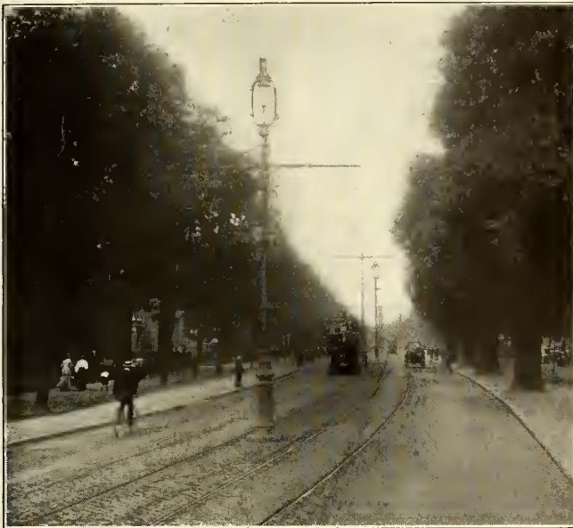
SOUTHAMPTON AVENUE WHERE THE JOINTS WERE INSTALLED
