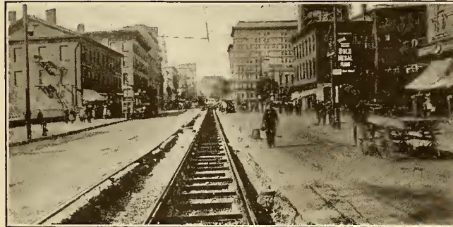
STEEL TIE CONSTRUCTION
