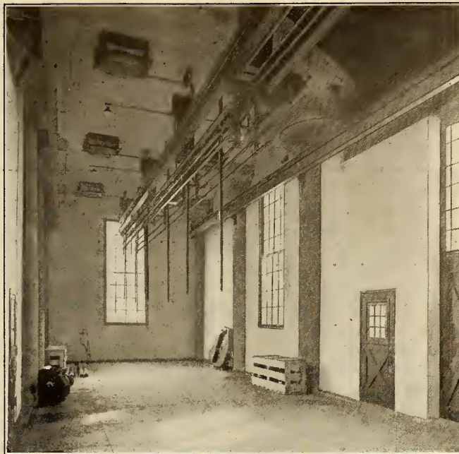
THE BOTTOM OF ONE OF THE CONCRETE BUNKERS SHOWING THE SIX DUPLEX GATES AND OPERATING LEVERS, AND THE LORRY RUNWAYS
