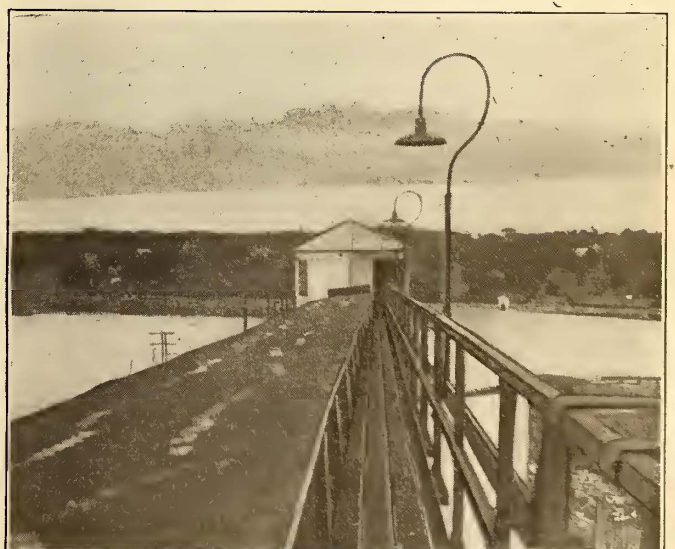
AT LEFT, LOOKING DOWN THE INCLINED CONVEYOR STRUCTURE—THE TRESTLE OVER THE CRUSHER IS SEEN AT THE RIGHT AND THE MAIN RIGHT-OF-WAY AT THE LEFT. AT RIGHT, THE CONVEYOR STRUCTURE BETWEEN BUNKERS, SHOWING THE MANNER IN WHICH COMMUNICATION BETWEEN CUPOLAS IS AFFORDED
