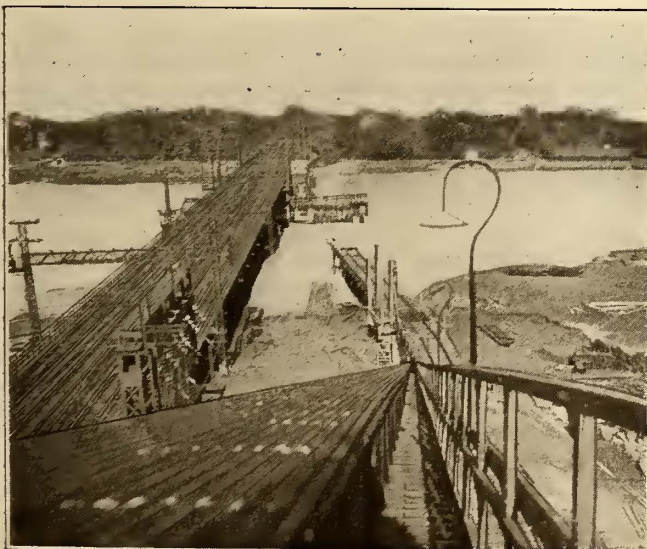
AT LEFT, LOOKING DOWN THE INCLINED CONVEYOR STRUCTURE—THE TRESTLE OVER THE CRUSHER IS SEEN AT THE RIGHT AND THE MAIN RIGHT-OF-WAY AT THE LEFT. AT RIGHT, THE CONVEYOR STRUCTURE BETWEEN BUNKERS, SHOWING THE MANNER IN WHICH COMMUNICATION BETWEEN CUPOLAS IS AFFORDED
