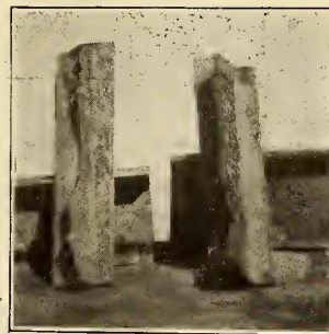
FIG. 4.—WHAT CORROSION DOES TO RAILS
