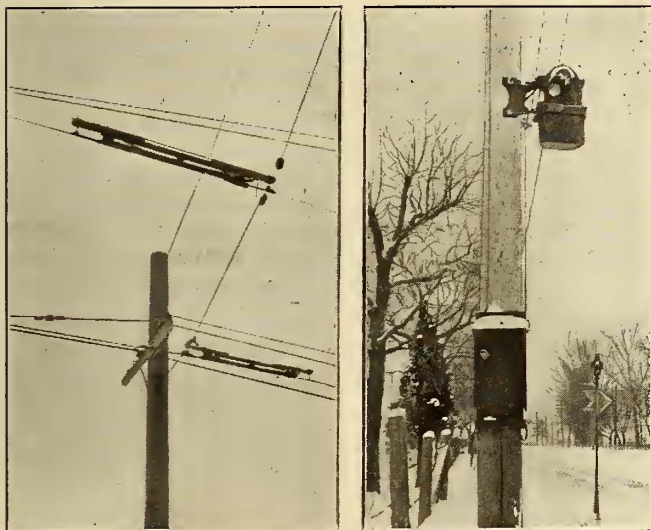
SIGNAL INSTALLATION AT WAUKESHA WEST LIMITS
