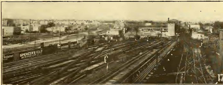
TEMPORARY CONSTRUCTION AT THE TERMINAL
