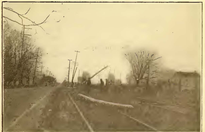
THESE PICTURES ILLUSTRATE A SURPRISINGLY CLEAN SWEEP OF TROLLEY POLES, WRECKAGE BEING CLEANED FROM RIGHT-OF-WAY AND NEW POLES ERECTED. POLES BELONGING TO OTHER UTILITIES CAUSED MUCH OF THE DAMAGE
