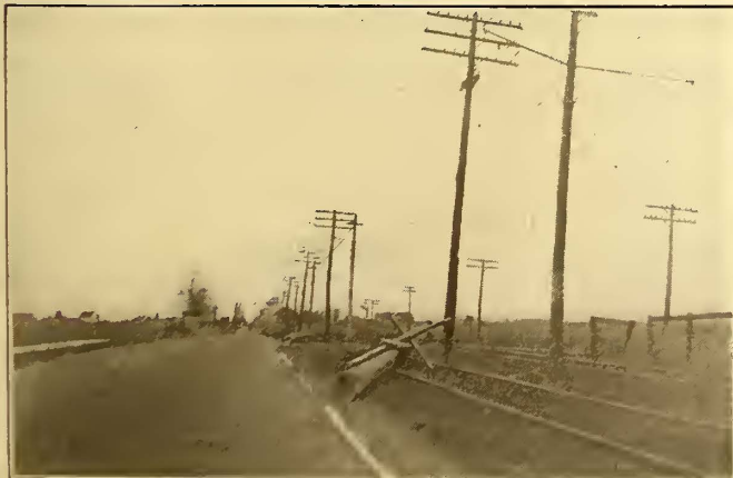
THESE PICTURES ILLUSTRATE A SURPRISINGLY CLEAN SWEEP OF TROLLEY POLES, WRECKAGE BEING CLEANED FROM RIGHT-OF-WAY AND NEW POLES ERECTED. POLES BELONGING TO OTHER UTILITIES CAUSED MUCH OF THE DAMAGE
