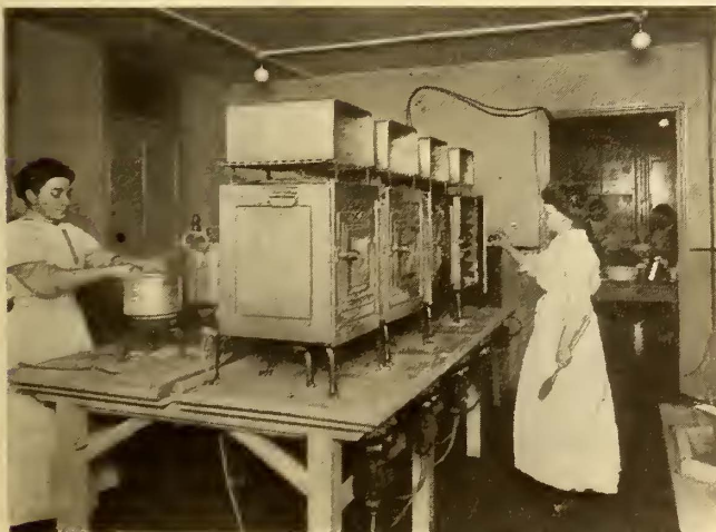
ELECTRIC COOKING KITCHEN OF UNDERGROUND FEMALE STAFF CLUB, EARL'S COURT
