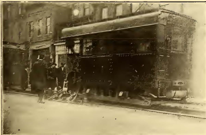
AT LEFT, WELDING CAR IN PLACE READY FOR OPERATION. AT RIGHT, CONNECTION FROM THE WELDING CAR TO THE TRACK EQUIPMENT
