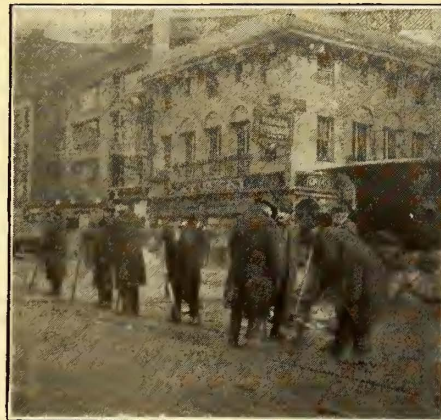
SNOW-FILLED CONDUIT, REMOVING ICE FROM TRACK AND STALLED CARS, NEW YORK RAILWAYS
