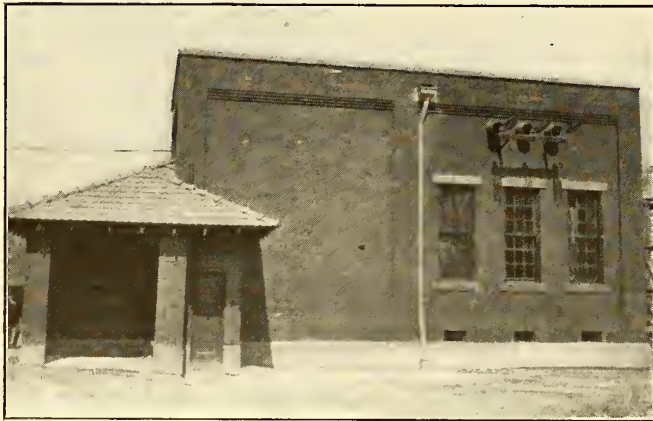
NOISELESS SUBSTATION SHOWING TRANSFORMER ROOM VENTILATION OPENINGS AT FLOOR LINE AND HIGH-TENSION LINE ENTERING AT CEILING
