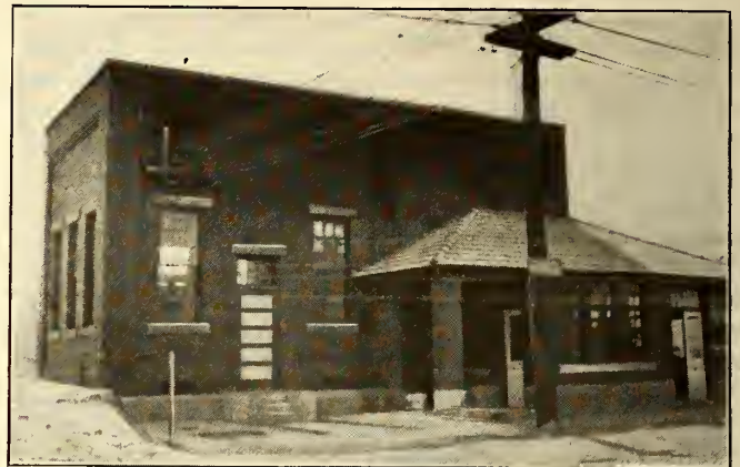
OPPOSITE SIDE OF SUBSTATION SHOWING OUTGOING FEEDER CABLES AND WAITING ROOM CONVERTED INTO CONFECTIONERY STORE
