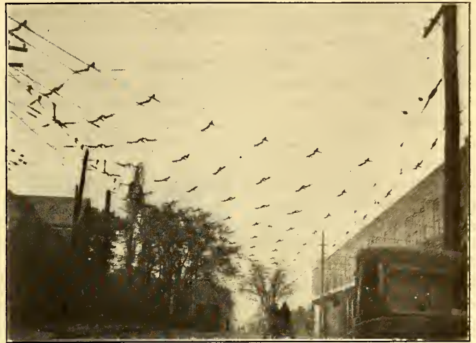
CROSS CATENARY SUPPORT FOR OVERHEAD, ALONG FRONT OF CARHOUSE CAN BE SEEN IN THIS VIEW OF "PERMANENT" OVERHEAD CONSTRUCTION
