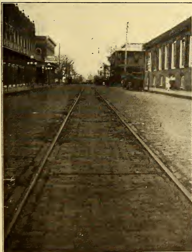
TYPICAL SURFACE APPEARANCE OF TAMPA'S TRACK AND BRICK PAVING
