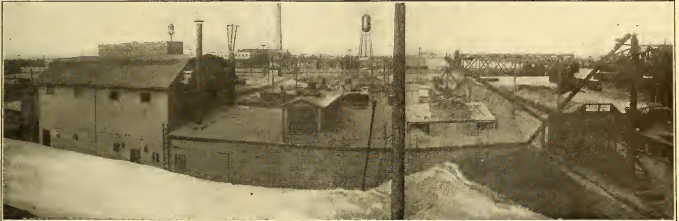
PANORAMIC VIEW OF PUBLIC SERVICE SAND PLANT
