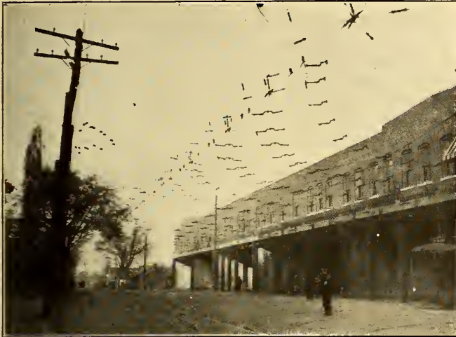
BACKBONE CONSTRUCTION ON CURVES AND CATENARY CONSTRUCTION OVER STRAIGHT TROLLEY IN FRONT OF ATLANTA CARHOUSE
