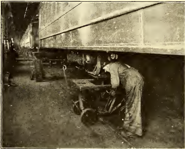
REMOVING A COMPRESSOR FROM THE CAR
