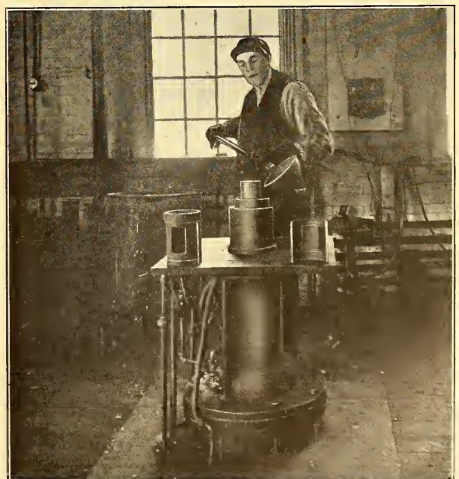
WITH THIS MACHINE ONE MAN CAN BABBITT 100 BEARINGS A DAY
