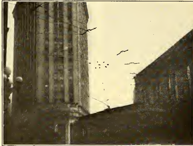
BACKBONE REINFORCEMENT OF TROLLEY CURVE AT BUSY DOWNTOWN CORNER WHERE ABSENCE OF ANCHOR POLES BROUGHT BULL-RING CONSTRUCTION INTO USE
