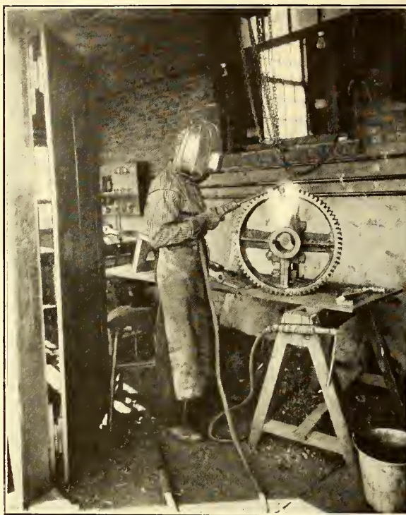
WELDING SPLIT GEAR INTO SOLID ONE
