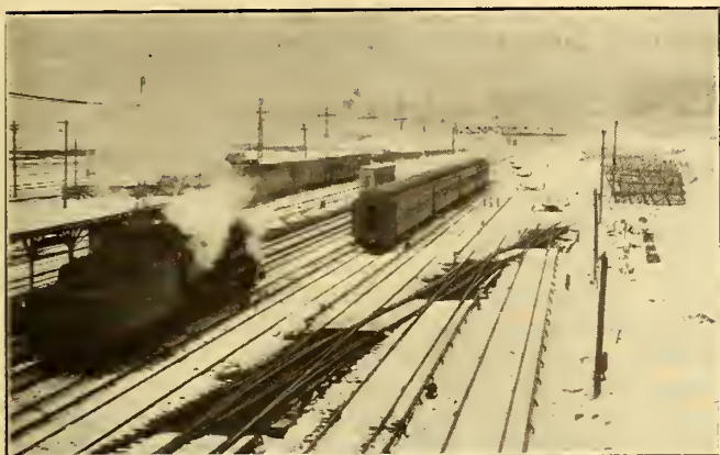
THIS ILLUSTRATES THE EFFECTIVENESS OF THE HEATERS AT HARMON, N. Y.
