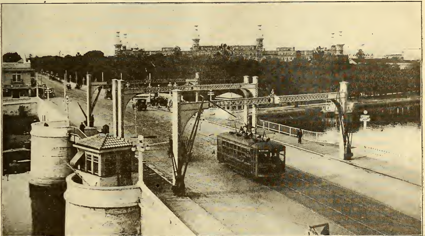
SAFETY CAR CROSSING DRAWBRIDGE IN TAMPA
