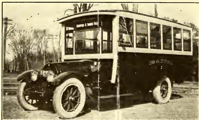
TYPE OF NINETEEN-SEAT CADILLAC MOTOR BUS USED. AT LEFT, SHOWING HOW BUSES ARE SIGNED. AT RIGHT, SHOWING ONE-MAN ENTRANCE AND EXIT
