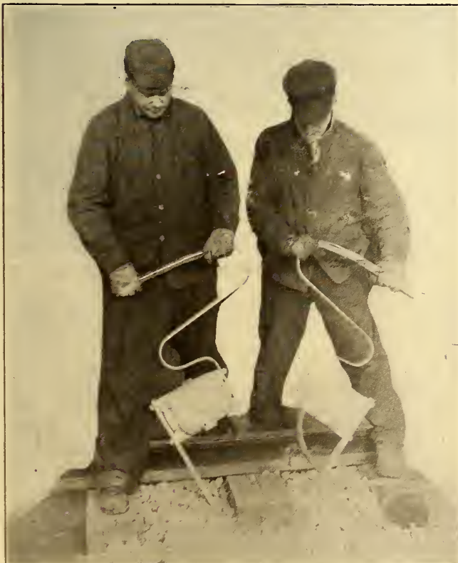
CENTRIFUGAL-ELECTRIC TIE TAMPER IN OPERATION
