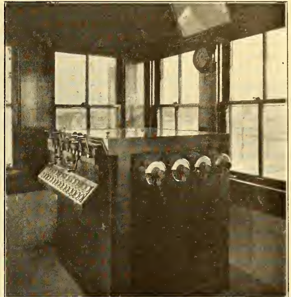
AT LEFT, SIGNAL TOWER AT CROSSING OF MAIN TRACK OF P. R. R. AND DOUBLE TRACK OF U. R. & E. CO. AT RIGHT, INTERLOCKING MACHINE IN SIGNAL TOWER
