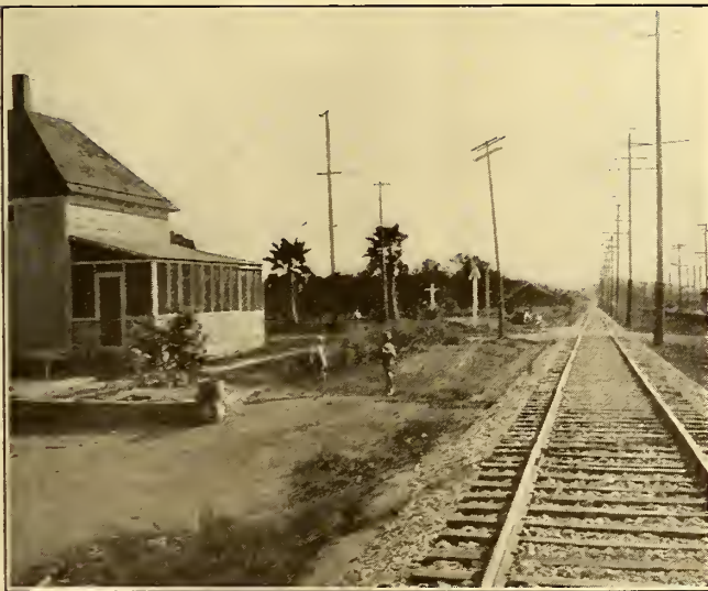
STANDARD TYPE OF GRADED AND OILED ROAD CROSSING BUILT BY PACIFIC ELECTRIC RAILWAY
