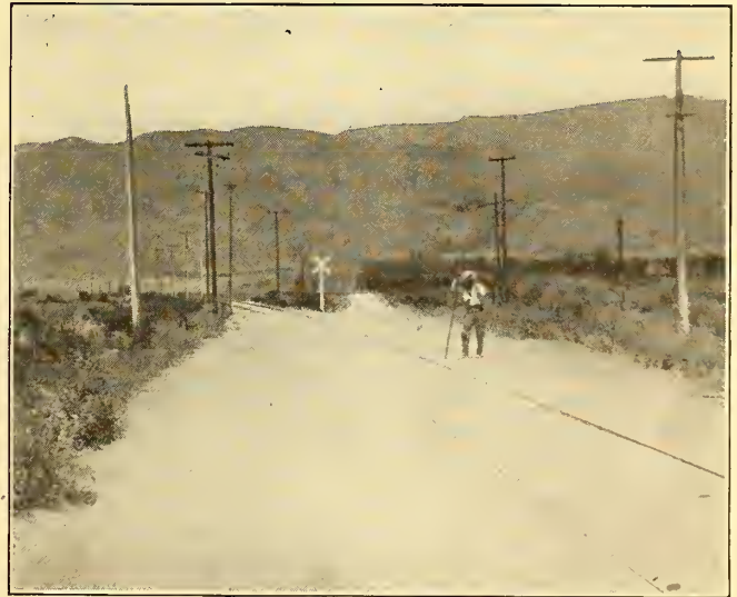
STANDARD TYPE OF GRAVELED ROAD CROSSING PRODUCED BY NATURAL SOIL CONDITIONS
