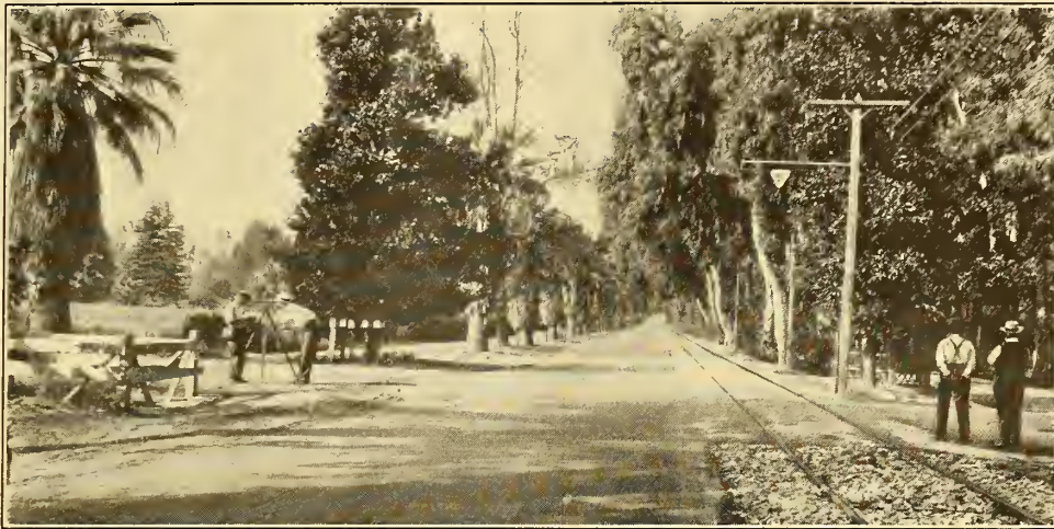
STANDARD TYPE OF OIL MACADAM ROAD CROSSING CONSTRUCTED BY PACIFIC ELECTRIC RAILWAY
