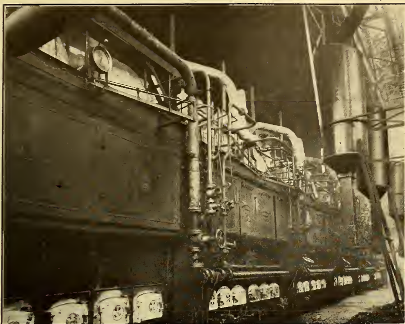
AT LEFT, LOWER FLOOR LEVEL IN BOILER PLANT, SHOWING HAND-FIRED BOILERS AND TEMPORARY COAL BUNKERS. AT RIGHT, FIRING AISLE IN THE NEW BOILER PLANT, SHOWING THE NEW UPPER OPERATING FLOOR LEVEL AND THE COAL BUNKERS FOR THE HAND-FIRED BOILERS ON THE LOWER FLOOR LEVEL
