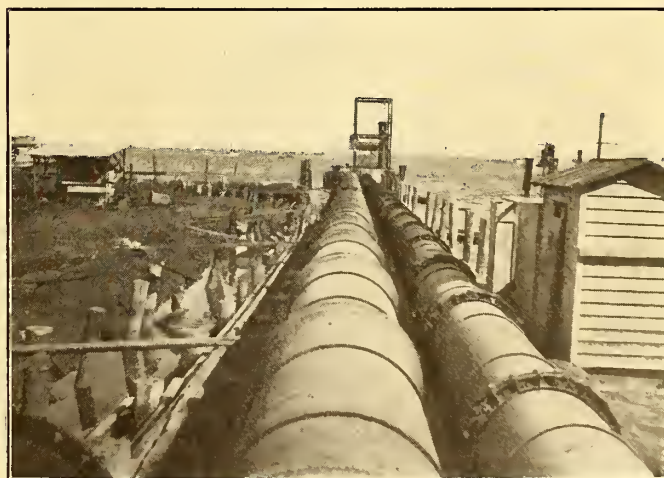
AT LEFT, CHAIN BUCKET COAL CONVEYOR AS IT PASSES OVER THE TOP OF THE BOILER HOUSE TO DISCHARGE IN THE OVERHEAD BUNKER. AT RIGHT, NEW AND OLD SIPHON PIPE LINES EXTENDING OUT INTO THE COOPER RIVER
