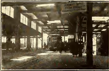
Andrew Square transfer station—surface to subway
