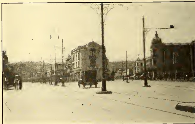
STREET SCENE IN VALPARAISO, CHILE, WITH STREET CARS DESTROYED
