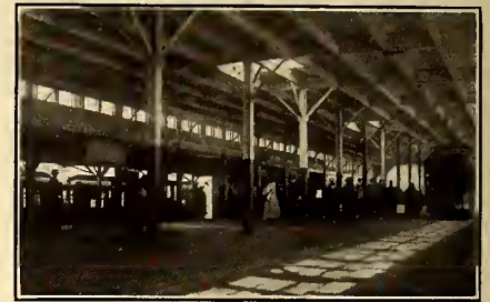
Everett Station—elevated train unloading
