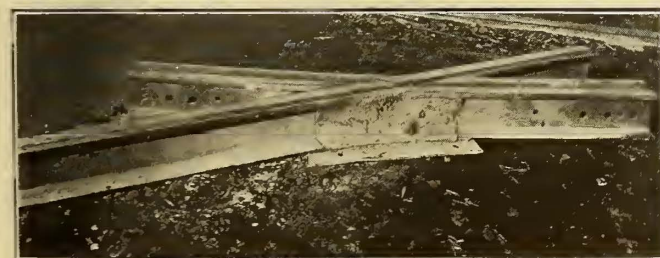
AT TOP, MANGANESE INLAID CROSSING REPLACED WITH THERMIT WELDED CROSSING. AT LEFT, THERMIT WELDED CROSSOVER WHICH REPLACED CAST MANGANESE INSERT AT ST. JOSEPH. AT RIGHT, THERMIT WELDED CROSSING FOR INTERSECTION WITH STEAM RAILROAD.
