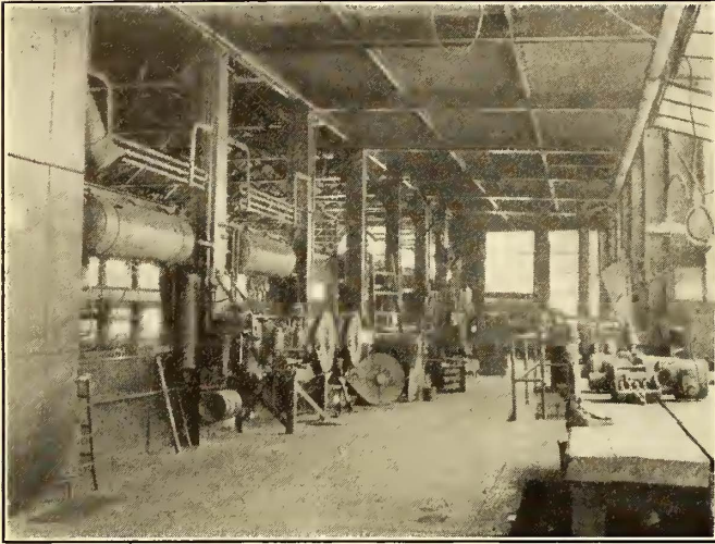
AT LEFT, THE AIR BRAKE DEPARTMENT IS LOCATED ON THE NORTH BALCONY. AT RIGHT, INTERIOR OF TWO-TRACK PAINT SHOP, SHOWING PERMANENT PLATFORMS AND RACKS FOR STORAGE OF SEAT CUSHIONS AND BACKS
