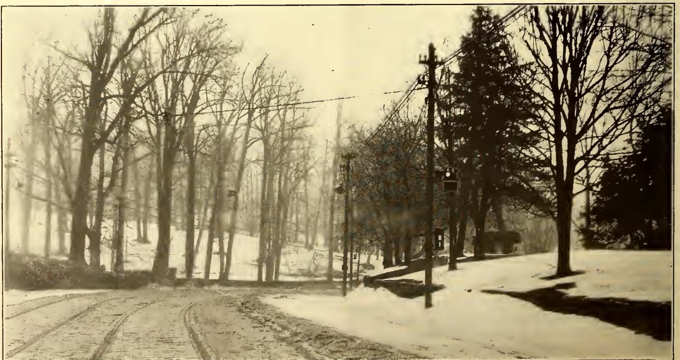
SIGNAL AND DOUBLE CONTACTOR PROTECTING REAR END. OGONTZ HILL
