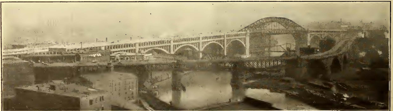
New High Level bridge spanning the Cuyahoga Valley, just west of the Public Square, Cleveland. In the foreground is the old Superior Viaduct. There were two tracks on the old viaduct, which were in the center of the roadway; there are four tracks
