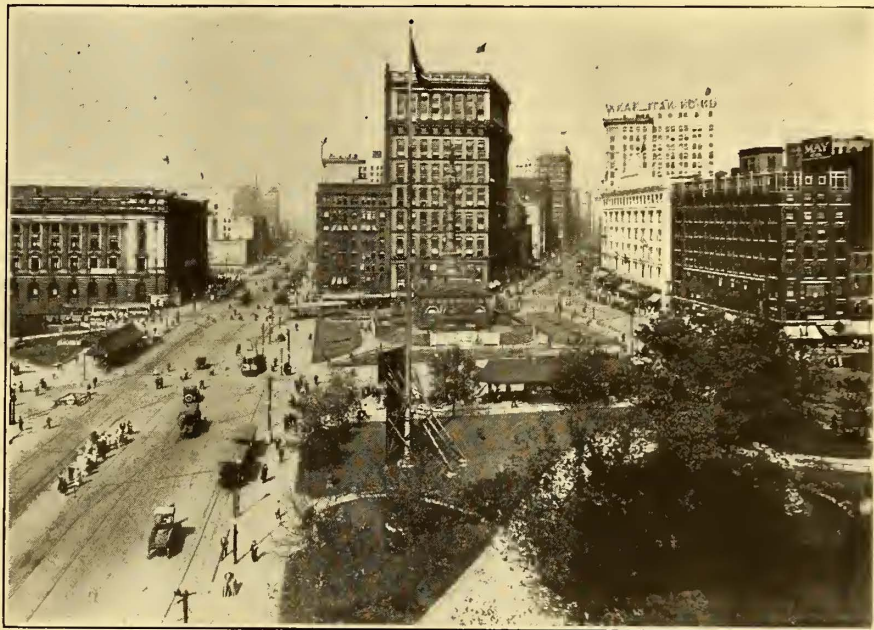
The Public Square, at Cleveland, showing “Monument” loop in exact center, “Federal Building” loop on the left, and the “Forest City” loop in direct foreground. Street shown at left center is Superior Avenue, widest of Cleveland's thoroughfares. Note six tracks are laid in this street and people waiting between tracks at loading station. Street at right center of picture is the world famous Euclid Avenue.
