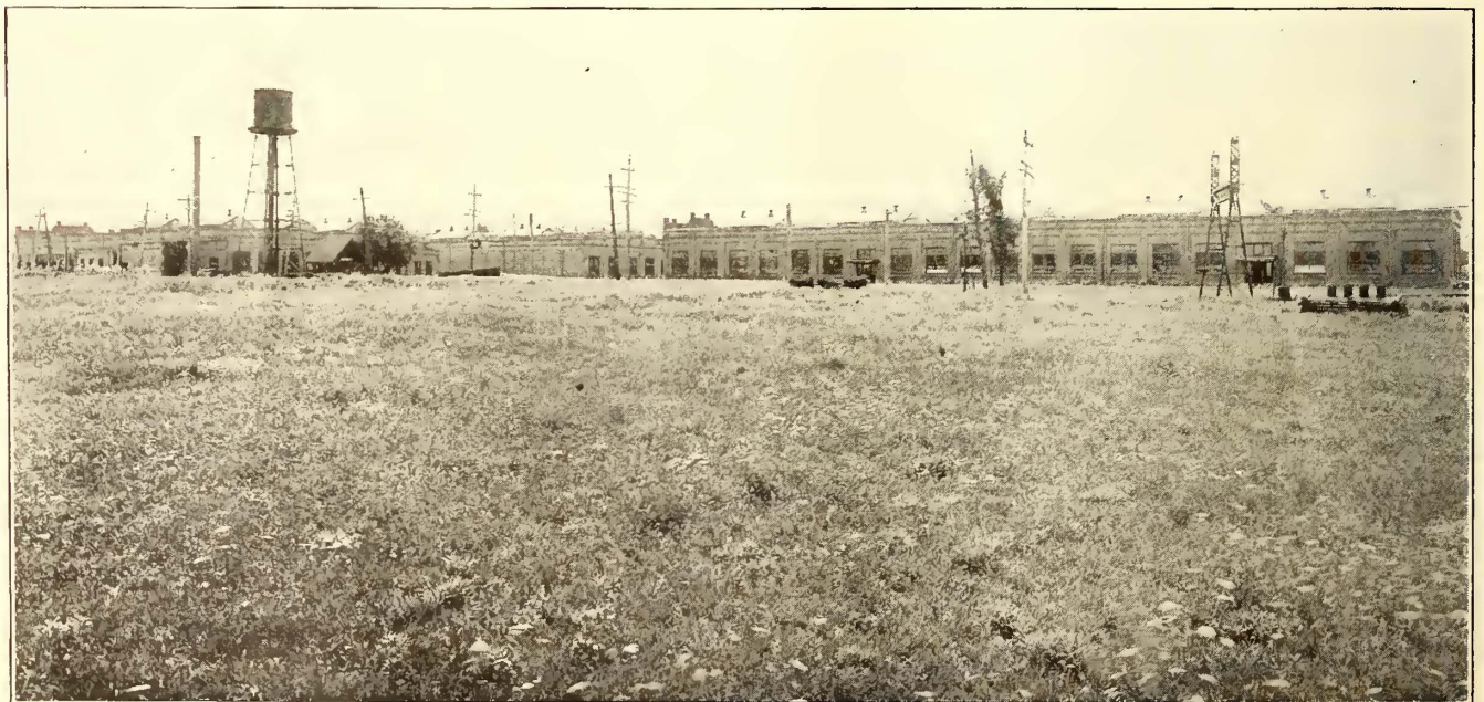
LEFT TO RIGHT—SHOP, CARHOUSE AND OFFICE BUILDING
