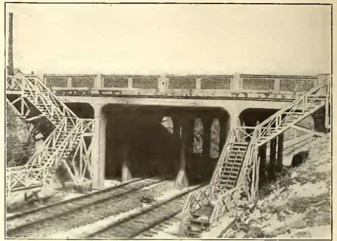
TYPICAL BRIDGE CONSTRUCTION, SHOWING PROVISION FOR AN ULTIMATE OF FOUR TRACKS, AND TEMPORARY STAIRS DOWN TO THE LOADING POINT
