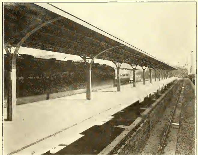
A VIEW SHOWING THE PITS AND PLATFORM CONSTRUCTION, ENABLING INSPECTORS TO PASS DIRECTLY FROM ONE PIT TO ANOTHER. THE SPACE BENEATH THE PLATFORM IS OPEN
