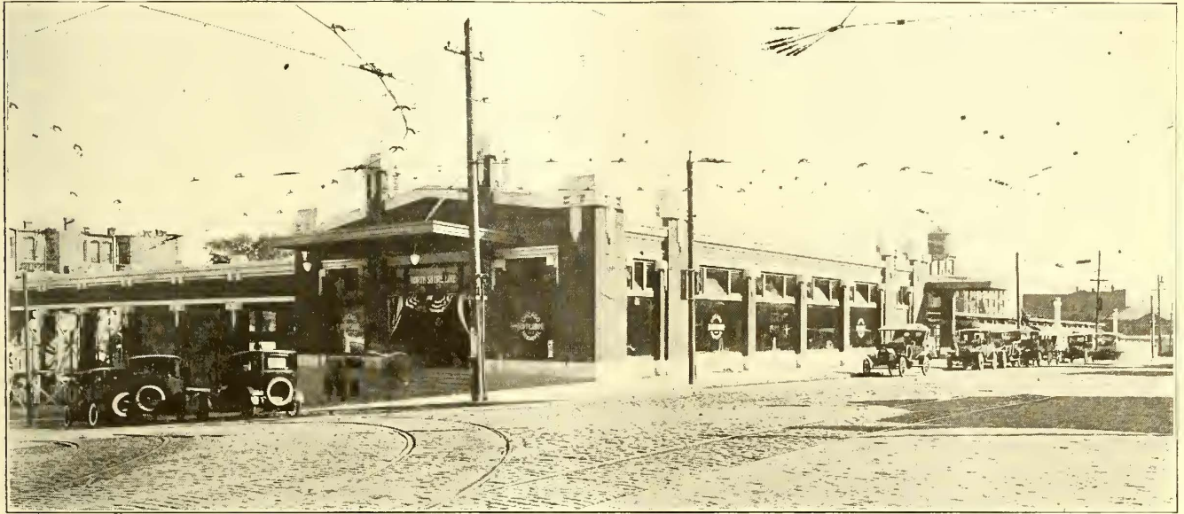
THE NEW MILWAUKEE TERMINAL FRONTS ON SYCAMORE STREET AT SIXTH AVENUE, THREE BLOCKS FROM THE HEART OF MILWAUKEE
