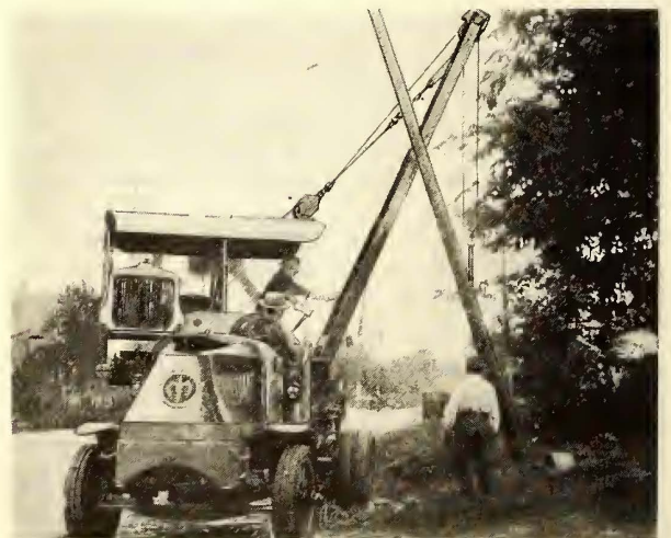
TRANSPORTING A POLE IS SIMPLE FOR THE CRANE AND SETTING IT IS JUST AS EASY
