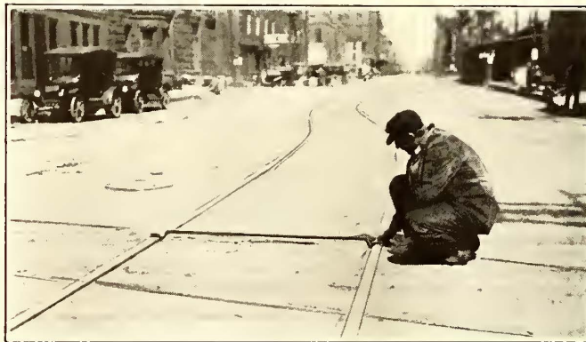
THE TEMPLATE IN USE ON THE TRACK
