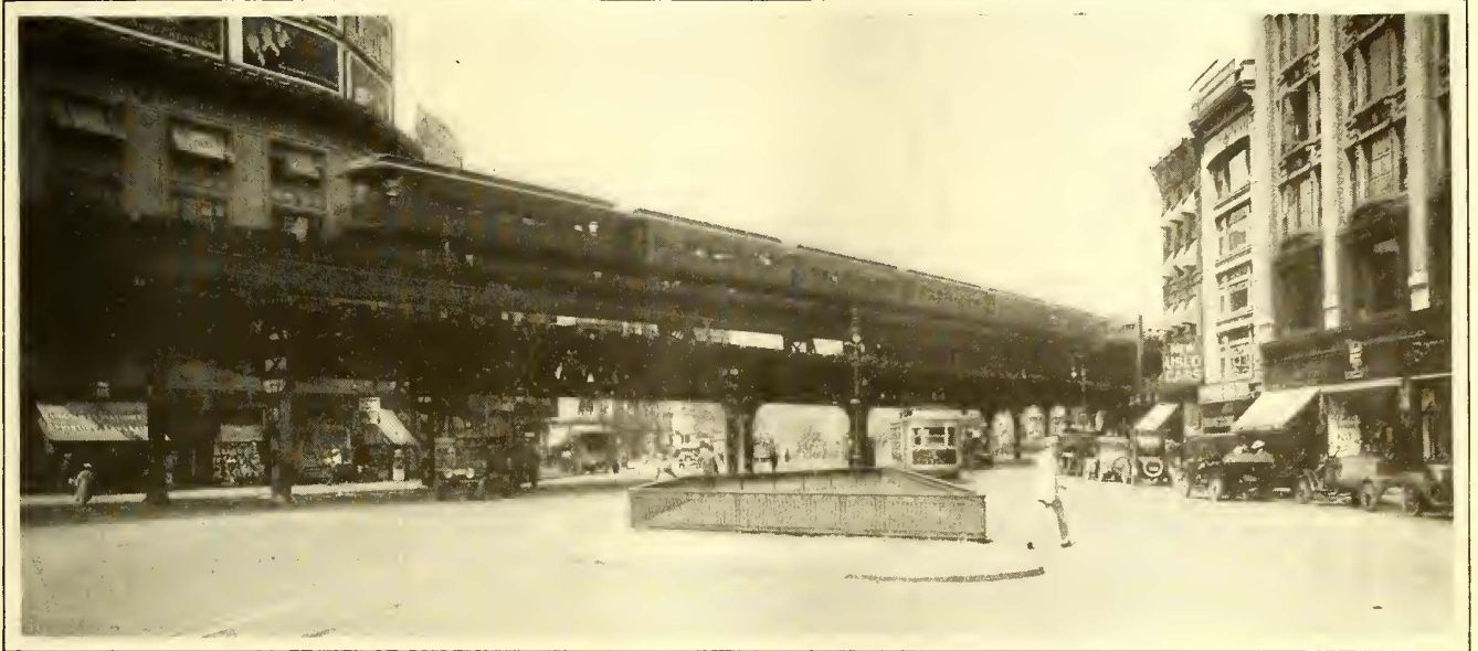
View on Broadway near Sixty-fifth Street, New York, where the Manhattan Elevated crosses the West Side division of the Interborough Subway
