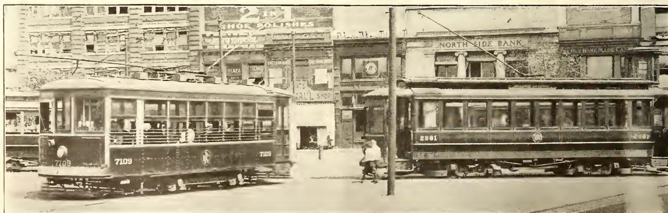
Cross-seat safety car and longitudinal-seat two-man car at Williamsburg Bridge Plaza, Brooklyn
