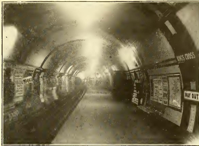
A deep-level Underground station, King's Cross on the Piccadilly line
