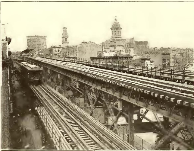
The completion of the third track on the Ninth Avenue line added greatly to the carrying capacity.
