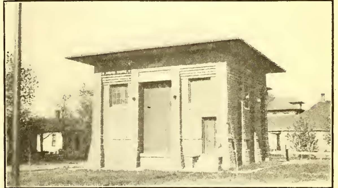
AUTOMATIC SUBSTATION IN COUNCIL BLUFFS, IOWA, BUILT OF OLD GRANITE PAVING BLOCKS
