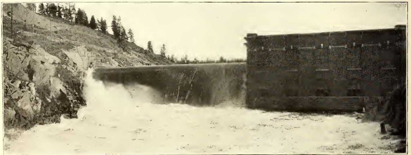
NINE-MILE BRIDGE HYDRAULIC PLANT SUPPLIES PART OF SPOKANE'S RAILWAY POWER
