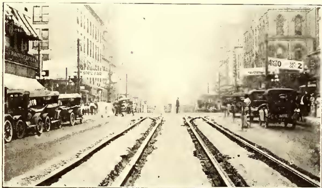
PAVEMENT CUT AWAY FROM TRACKS TO ALLOW REPLACEMENT OF RAILS
