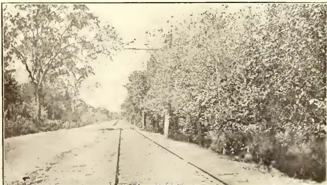
BROCKTON-EASTON LINE RAISED FROM 6 IN. TO 2 FT. AND REBALLASTED
