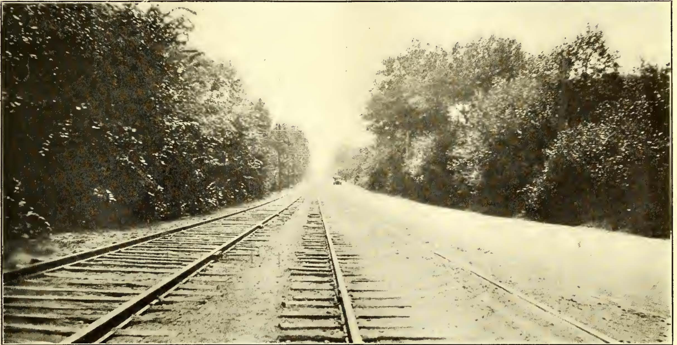
DOUBLE TRACK LINE RAISED FROM 8 IN. TO 14 IN. TO PROVIDE BETTER DRAINAGE
