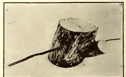
UNUSUAL CONDITION FOUND ON DISTRIBUTION SYSTEM
