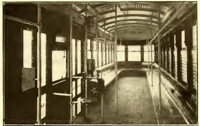
CONDUCTOR'S STATION IN NEW PUBLIC SERVICE TRAIL CAR
