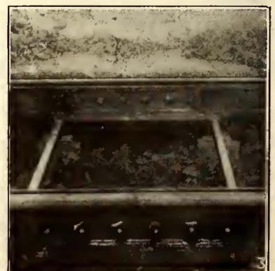
1—DEFLECTOR BAR IN POSITION FOR WELDING TOP EDGE OF PLATES. 2—THE WELDER AT WORK. 3—FINISHED WELDED JOINT, TOP AND BOTTOM SEAMS AND ENDS OF BOLTS WELDED, RAILS SPOT WELDED TO TIES
