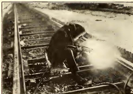
1—DEFLECTOR BAR IN POSITION FOR WELDING TOP EDGE OF PLATES. 2—THE WELDER AT WORK. 3—FINISHED WELDED JOINT, TOP AND BOTTOM SEAMS AND ENDS OF BOLTS WELDED, RAILS SPOT WELDED TO TIES
