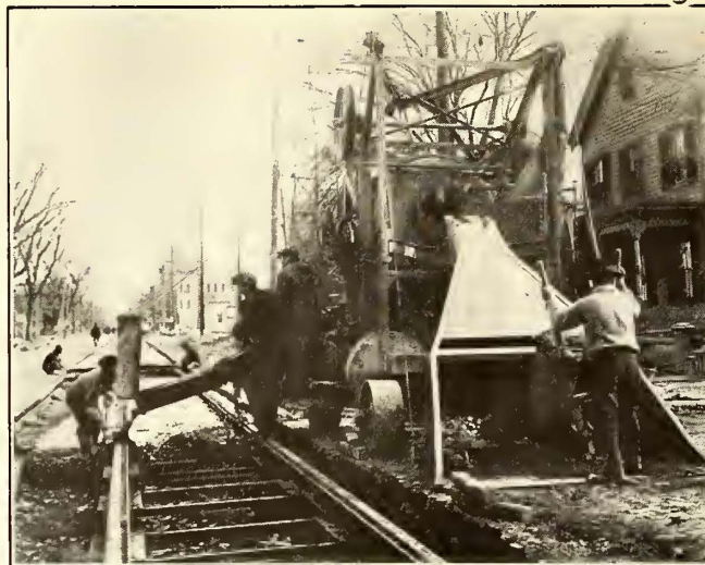
TYPE OF CONSTRUCTION USED ON MAIN STREET
