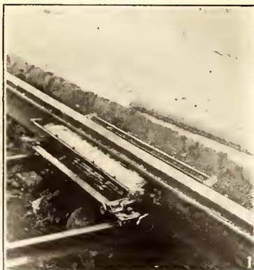
1—DEFLECTOR BAR IN POSITION FOR WELDING TOP EDGE OF PLATES. 2—THE WELDER AT WORK. 3—FINISHED WELDED JOINT, TOP AND BOTTOM SEAMS AND ENDS OF BOLTS WELDED, RAILS SPOT WELDED TO TIES
