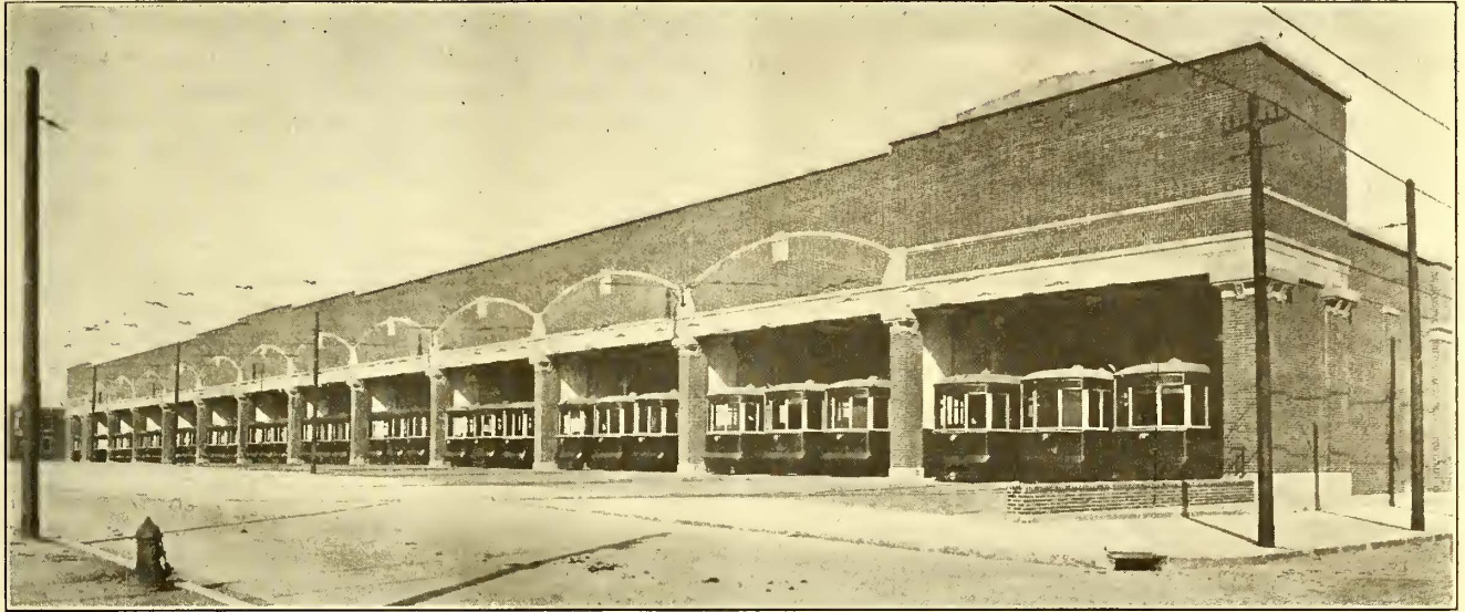
ALLOWHILL DEPOT, PHILADELPHIA RAPID TRANSIT COMPANY
