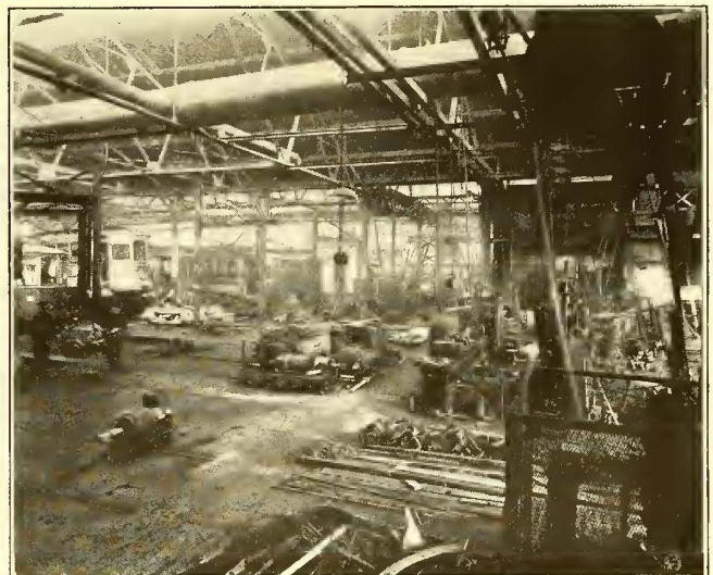
TYPICAL SHOP INTERIOR, PUBLIC SERVICE RAILWAY, CAMDEN
