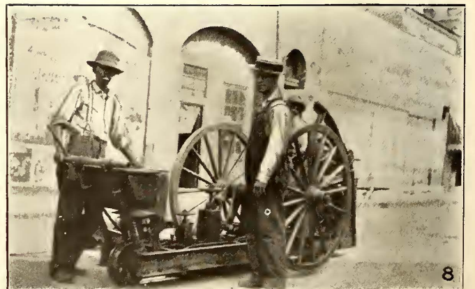
5—Repair to crossing by arc welding. 6—Dynamotor type arc-welding machine. 7—Seam-welded joint on 7-in. groove girder rail. 8—Reciprocating rail grinder.
