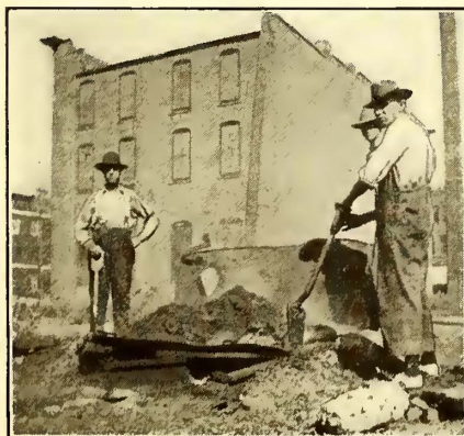
AT LEFT, HOW THE OLD ASPHALT PAVEMENT WAS MELTED UP. IN CENTER, PAINTING THE OPENING IN THE PAVEMENT WITH HOT TARVIA AS A BINDER BETWEEN THE ASPHALT AND CONCRETE. AT RIGHT, METHOD OF HAULING AND SPREADING THE ASPHALT TO FILL THE OPENINGS
