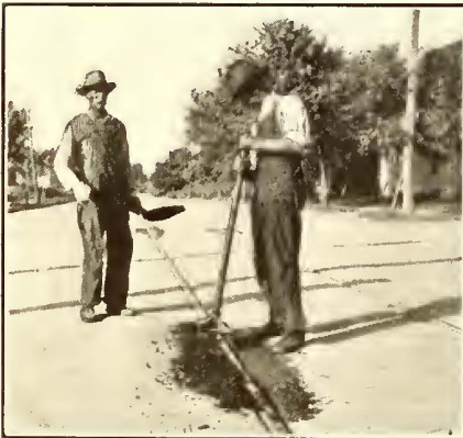
AT LEFT, TAMPING THE ASPHALT SOLID INTO THE OPENING. CENTER AND RIGHT, A WORK CAR, EQUIPPED WITH SIDE OUTRIGGER TO DRAG PLOW, FACILITATES EXCAVATION FOR NEW TRACK
