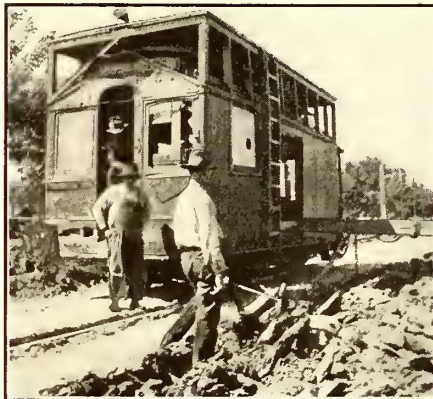
AT LEFT, TAMPING THE ASPHALT SOLID INTO THE OPENING. CENTER AND RIGHT, A WORK CAR, EQUIPPED WITH SIDE OUTRIGGER TO DRAG PLOW, FACILITATES EXCAVATION FOR NEW TRACK
