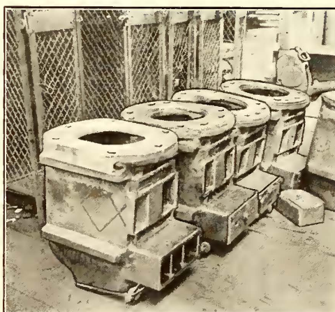
JOURNAL BOXES WITH NEW WEARING PLATES IN POSITION
