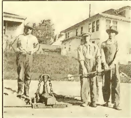
AT LEFT, OPENING IN CONCRETE PAVING MADE IN ORDER TO REPAIR JOINTS. IN CENTER, HEAVY CHAIN AND RAIL GRIPS USED IN LIFTING LOW JOINTS. AT RIGHT, CHAIN AND JACK ASSEMBLY IN POSITION TO LIFT RAILS
