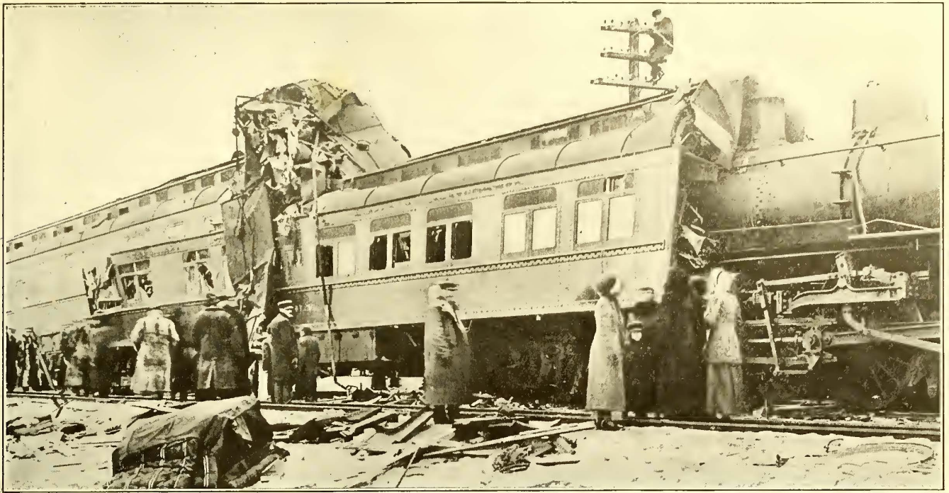
THE PENETRATION OF THE LOCOMOTIVE SELDOM EXTENDS THE DEPTH OF THE VESTIBULE. THE GREATEST DAMAGE OCCURS WHERE ONE CAR OVER-RIDES ANOTHER
