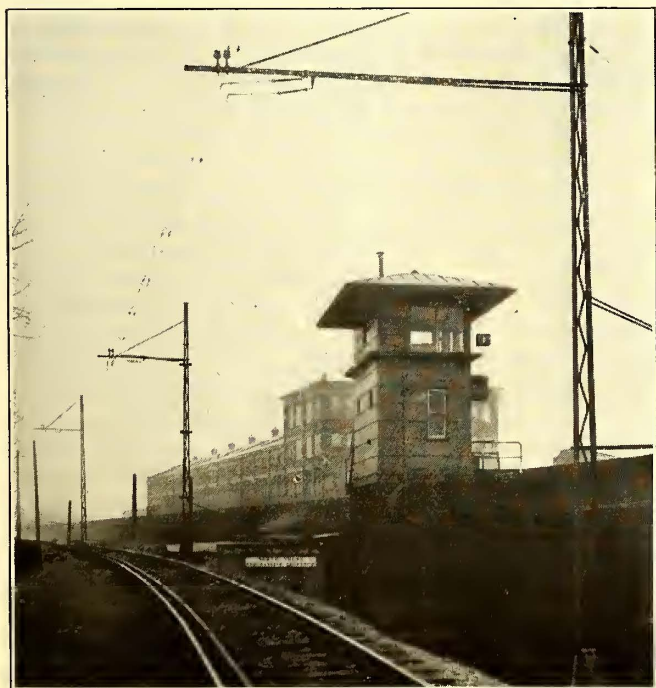
DOUBLE TROLLEY WAS INSTALLED OVER THE GRADE UP TO THE ELEVATED TRACK—SIMPLE SINGLE-TRACK POLE AND MAST-ARM CONSTRUCTION
