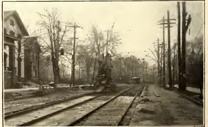
AT LEFT, TIES IN PLACE AND TRACK CONSTRUCTION STARTED. SUB-BASE COVERED WITH MANURE TO PREVENT FREEZING. AT RIGHT, TRACKS IN PLACE AND CONCRETE BEING POURED
