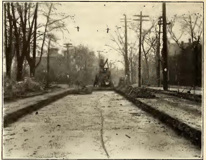
FOUNDATION READY FOR THE LAYING OF THE TRACKS
