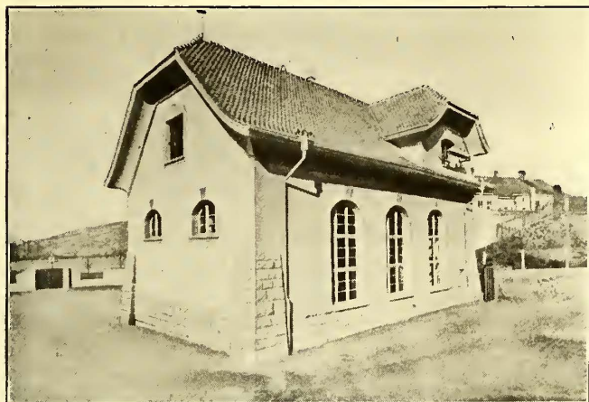
RIEHEN AUTOMATIC SUBSTATION, NEAR BASEL
