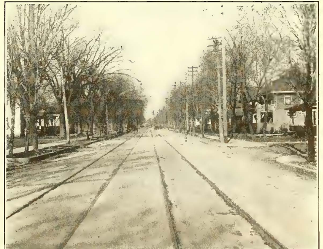
AT LEFT, TRACK CONSTRUCTION BLOCKED UP TO GRADE, SHOWING MECHANICAL TIES IN PLACE READY FOR POURING CONCRETE BASE AND PAVING, AND, AT RIGHT, APPEARANCE OF COMPLETED CONSTRUCTION
