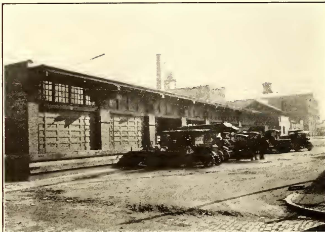
RECEIVING SIDE OF THE NEW TERMINAL
