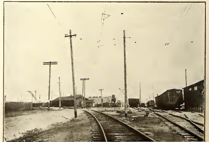
TWO VIEWS ON THE RIGHT-OF-WAY SHOWING OVERHEAD CONSTRUCTION ON CURVES AND GIVING SOME IDEA OF THE NATURE OF THE LINE
