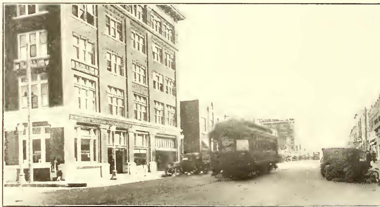
MAIN STREET, MIAMI, SHOWING CATENARY OVERHEAD WITH CONCRETE POLE CONSTRUCTION
