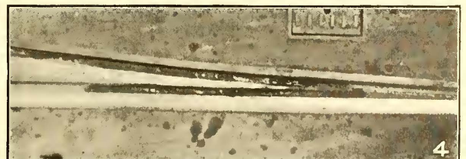
NO. 1—HOLE BROKEN THROUGH CAST-STEEL MATE IN DALLAS. NO. 2—APPEARANCE AFTER HOLE HAD BEEN FILLED WITH SOFT METAL. NO. 3—APPEARANCE AFTER THE MATE POINT HAD BEEN FORMED AND WELDING COMPLETED. NO. 4—THE COMPLETED JOB AFTER GRINDING
