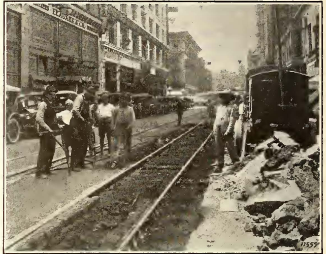
REMOVING PAVEMENT ALONG RAILWAY TRACK
