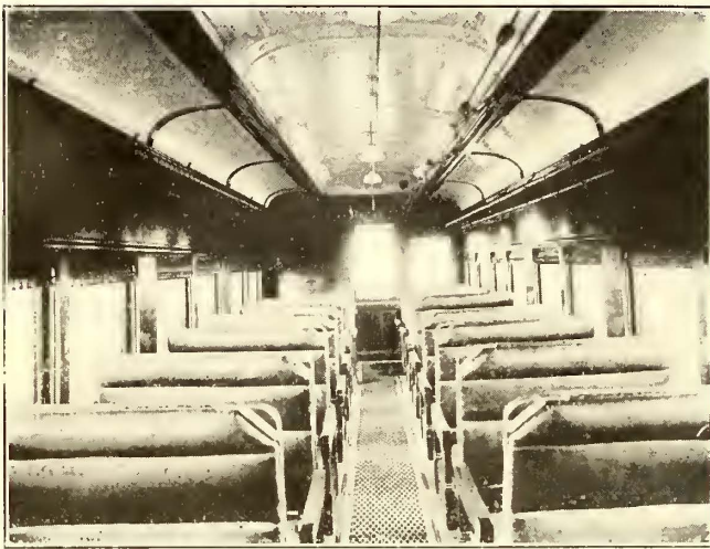
INTERIOR OF REBUILT TRAILER WAS FINISHED IN PLEASING WAY
