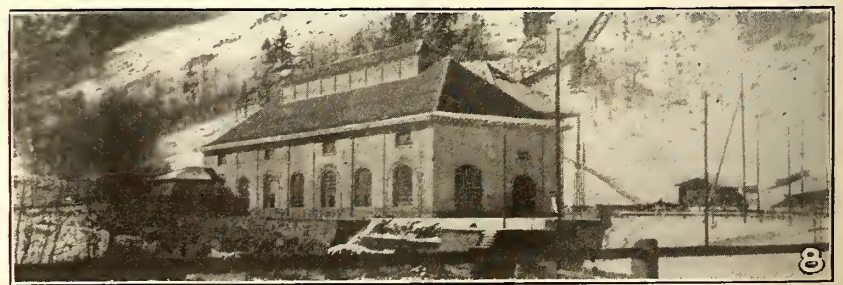
5—15,000-volt, single-phase locomotive and yards at Spiez, Lötschberg Railway. 6—11,000-volt, single-phase trolley construction at station, Rätische Bahn. 7—15,000-volt, single-phase trolley construction at Biasca, St. Gotthard Line. 8—Hydraulic power plant at Kandergrund, which under 985-ft. head generates 15,000-volt, 15-cycle, single-phase power.
