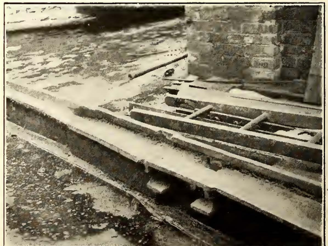
PIECE OF SPECIAL TRACKWORK REPAIRED BY ELECTRIC WELDING
