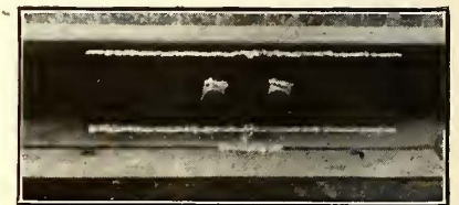
APPEARANCE OF COMPLETED JOINT AFTER WELDING
