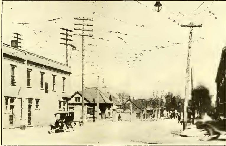
TYPICAL APPEARANCE OF THE OVERHEAD AT SPECIAL WORK LOCATION, SHOWING BACKBONE CONSTRUCTION
