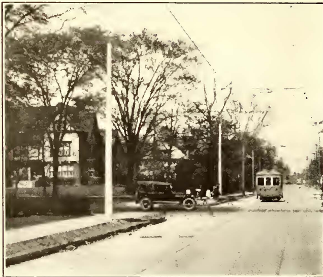
ANOTHER VIEW OF THE FINISHED TRACK AND OVERHEAD SHOWING SAFETY STOP SIGNS EMPLOYED AND CONCRETE POLES ERECTED ADJACENT TO BOULEVARDS
