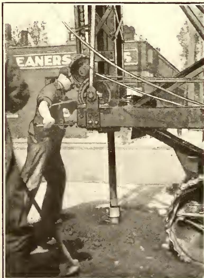
AT LEFT, DIGGING A POLE HOLE. THE AUGER IS ROTATED AND FORCED DOWNWARD. IN CENTER, ROTATION STOPPED AND AUGER BEING RAISED TO LIFT SOIL OUT OF THE HOLE. AT RIGHT, SPINNING AUGER TO REMOVE SOIL WHICH IS THROWN AROUND THE OUTSIDE OF THE HOLE
