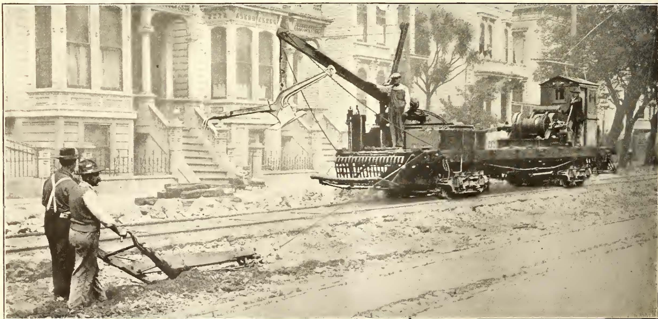
PLOW IN OPERATION—SPARE PLOW SUSPENDED FROM DERRICK WINCH ON THE PLOW CAR
