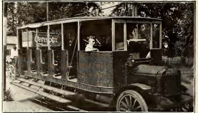
A GREAT SCHEME FOR FAST LOADING AND UNLOADING BUT REQUIRING TWO MEN. THE STEPS FOLD UP WHEN THE DRIVER PULLS THE ROPE
