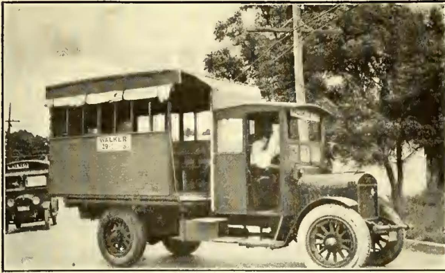
A FIELD REAL ESTATE OFFICE LIFTED ON THE TRUCK TO MAKE A BUS BODY. AFFECTIONATELY NAMED THE "GRAINARY"
