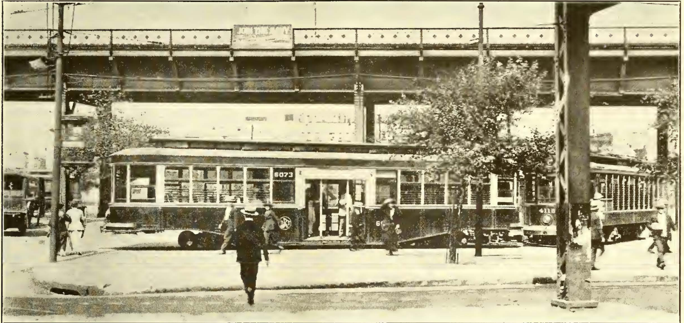
MOTOR AND TRAILER OPERATION IN BROOKLYN
