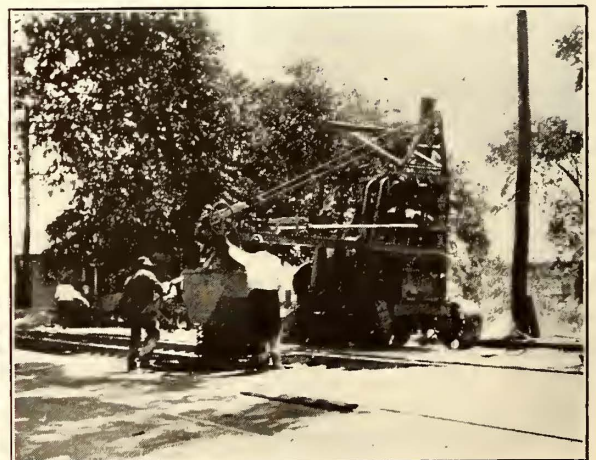
THE FIRST VIEW SHOWS THE COMPLETED TRACK READY FOR CONCRETE PAVEMENT—THE CONCRETE MIXER IN OPERATION IS SHOWN IN THE SECOND VIEW
