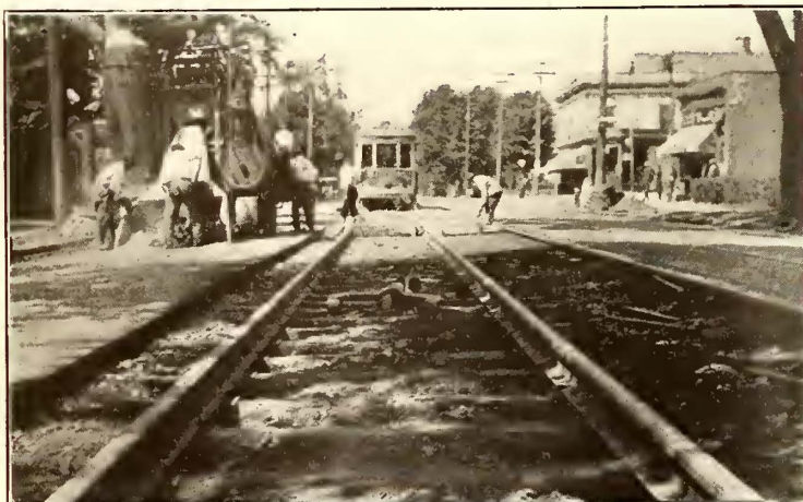
THE FIRST VIEW SHOWS THE COMPLETED TRACK READY FOR CONCRETE PAVEMENT—THE CONCRETE MIXER IN OPERATION IS SHOWN IN THE SECOND VIEW
