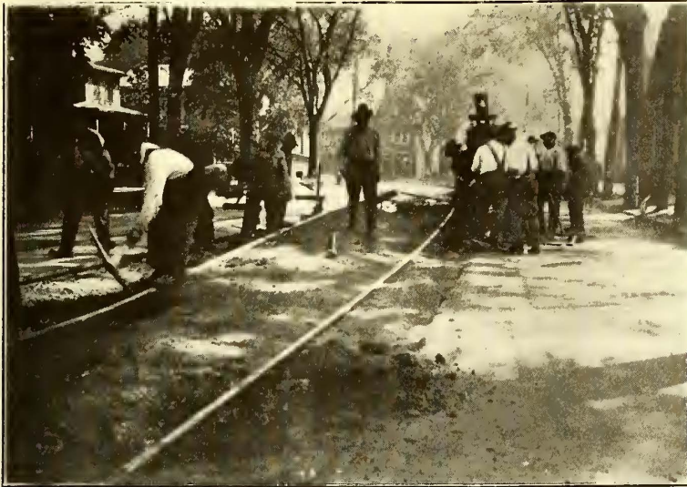
JACKING OLD TRACK OUT OF THE STREET—WHEN JACKED OUT THE STEAM SHOVEL LOADS THE SURPLUS MATERIAL ONTO TRUCKS
