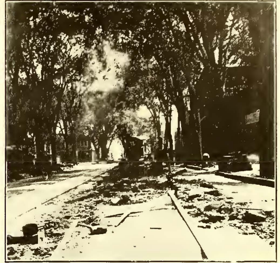
JACKING OLD TRACK OUT OF THE STREET—WHEN JACKED OUT THE STEAM SHOVEL LOADS THE SURPLUS MATERIAL ONTO TRUCKS
