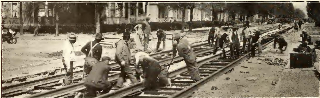
Installation of Steel Ties in Detroit
