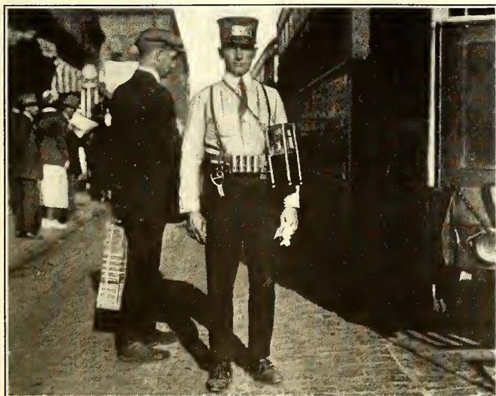
Street Collectors Are Supplied with a Belt-Type or Tripod-Type Farebox for Use in Front-End Collection in Congested Districts
