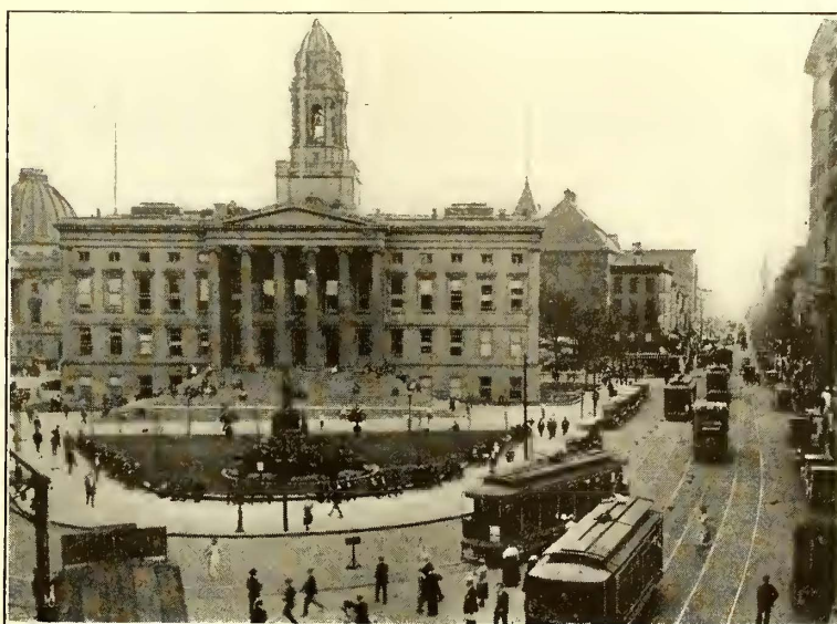
Borough Hall, Brooklyn, Showing Loop and How Study Has Resulted in Elimination of Congestion Due to a More Even Car Flow
