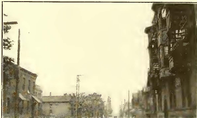
AN INSTANCE OF OVERHEAD CONSTRUCTION USED WHERE BUILDING WAS TOO CLOSE TO CURB TO SET POLE
