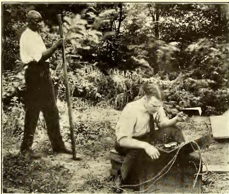
NEW EARTH CURRENT METER IN USE IN THE FIELD
